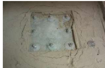
Fig 6: General view of the reinforced base after the test
