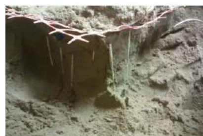
Fig 7: Sectional view of the reinforced base after the test
