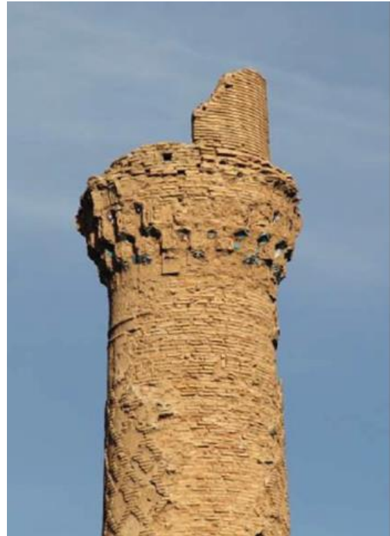
Fig 10: The minaret of Goharshad Begum School, Herat.
