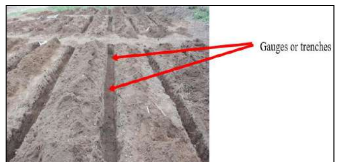
Fig 1: Staking and construction of the trenches (length: 4 m; width: 0.2 m; depth: 0.2 m and distance between two trenches: 1m)
