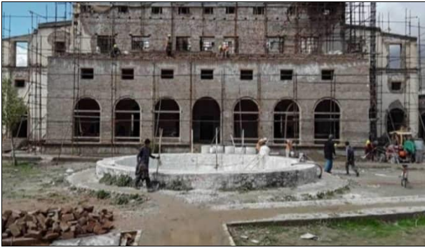
Fig 4: Front view of the before during reconstruction, Source: Authors
